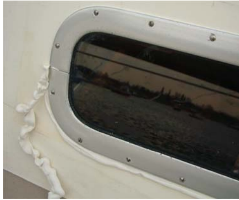
Figure 14: Trimming Surplus Window Sealant
